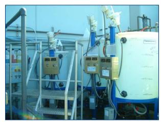
• Each pump comes with a special motor controller and encoder for controlling chemical dose rates into the GEM System. In order to set the dose rate, plant operations simply set the milliliters per minute via up and down arrows on the control panel interface.
