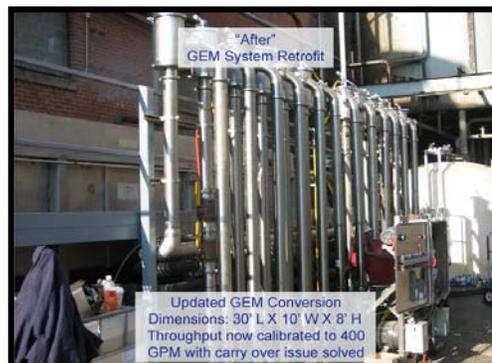
Two banks of model 300/600 LSGM's were chosen for this application due to varying flows throughout the day. Based upon the level of influent into the LSGM Heads, the second set of heads were provided to initiate when flow is at high/high, based upon level sensors in the
