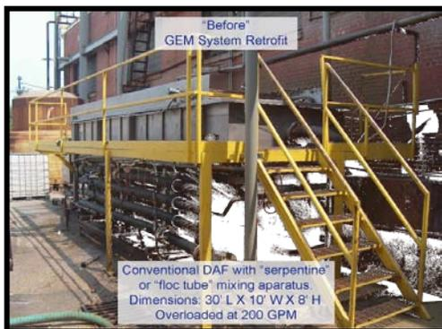
The existing Dissolved Air Flotation (DAF) unit was 30' long by 10' wide by 8' tall and equipped with "serpentine" (aka "floc tube") mixing apparatus. The floc tubes clogged on a regular basis making the existing system inefficient and labor-intensive.
