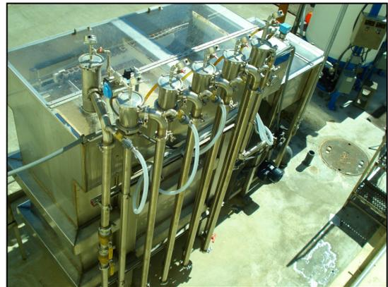
The equalization limitation also created a challenge in effectively treating load variances. A system that could adjust "Real Time" to follow TSS, FOG, and COD/BOD fluctuations was required. Since the LSGM technology is based on the "insitu" treatment principal, reaction times from chemical adjustments occur within seconds rather than minutes or hours. This enables the Client to effectively maximize reduction rates allowing the GEM System to accommodate inadequate equalization scenarios.
