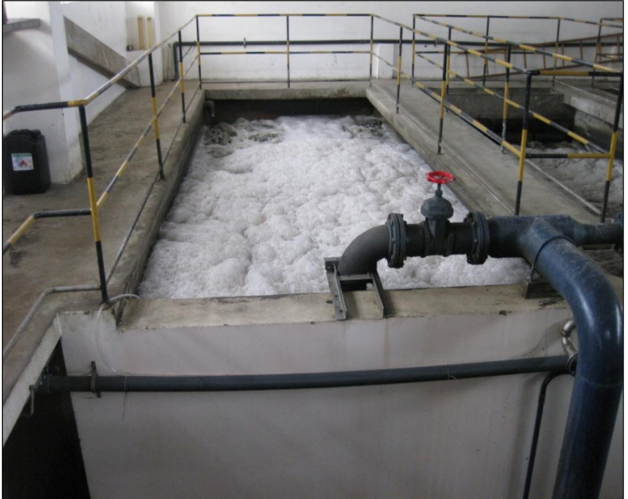
**Figure 1. Aeration tank of the MBBR System**
