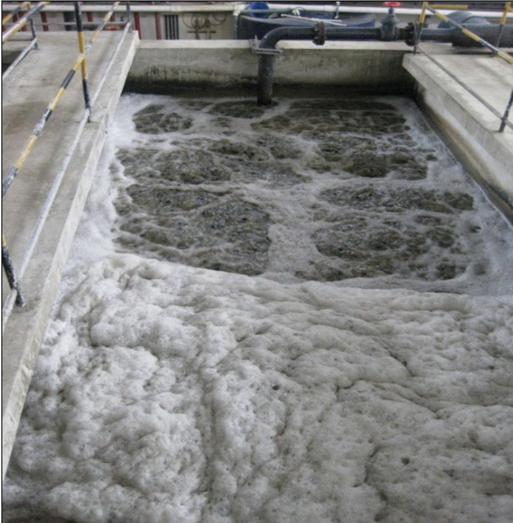
**Figure 2. Second aeration tank of the MBBR System**
